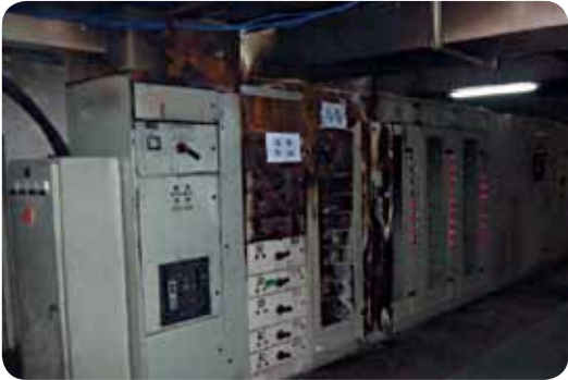
电容器过热引发的配电柜火灾事故照片 LV switchboard after a fire accident caused by capacitors' overheating
