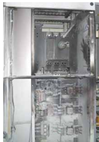
电容补偿柜事故照片 Capacitor bank after an accident
