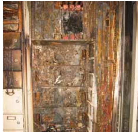
电容器过热引发的配电柜火灾事故照片 LV switchboard after a fire accident caused by capacitors' overheating
