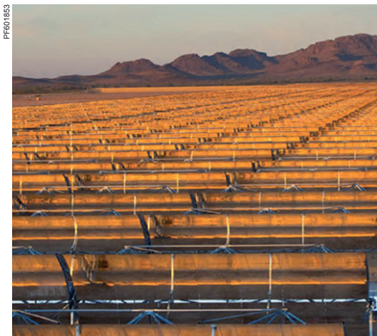
Parabolic trough application
